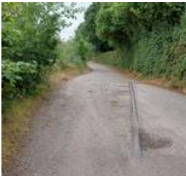
Photo 17 – Remains of railway track at Arpley Landfill (centre of road)
