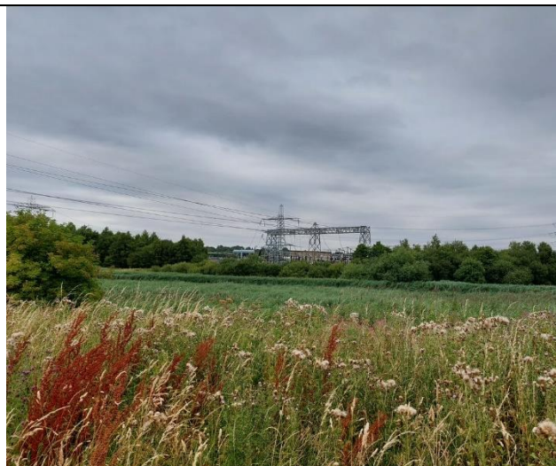
Photo 34 – Electricity substation between Rocksavage and Runcorn HAGIs
