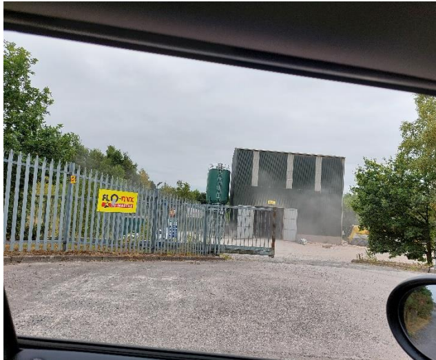
Photo 19 – FloMix UK in footprint of former timber yards and railway sidings along St Helens Canal.
