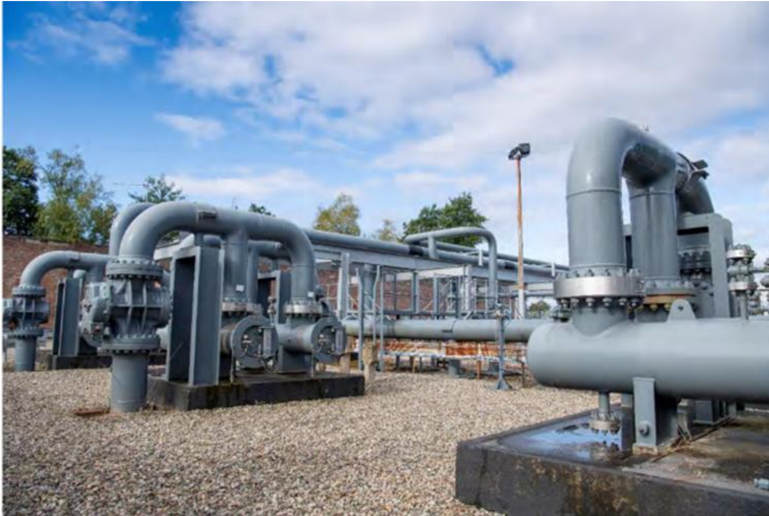
Figure 1.4 Photo of a methane Above Ground Installation
